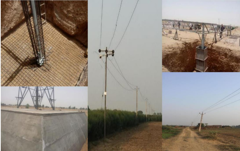
SMSA (Raj. Govt.) Building Work Alwar FY 2022-23
