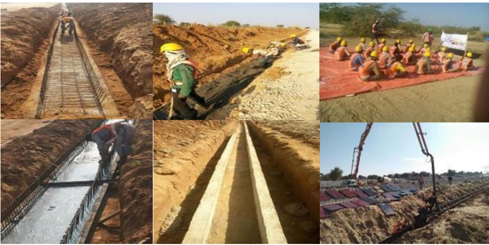
GR Infraprojects Ltd Construction of Embankment MP - morena FY 2017-18
