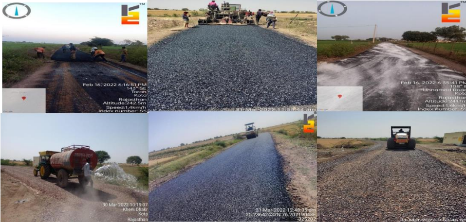
Larsen & Toubro Structure Work Bhagega-Shri madhopur FY 2016-17
